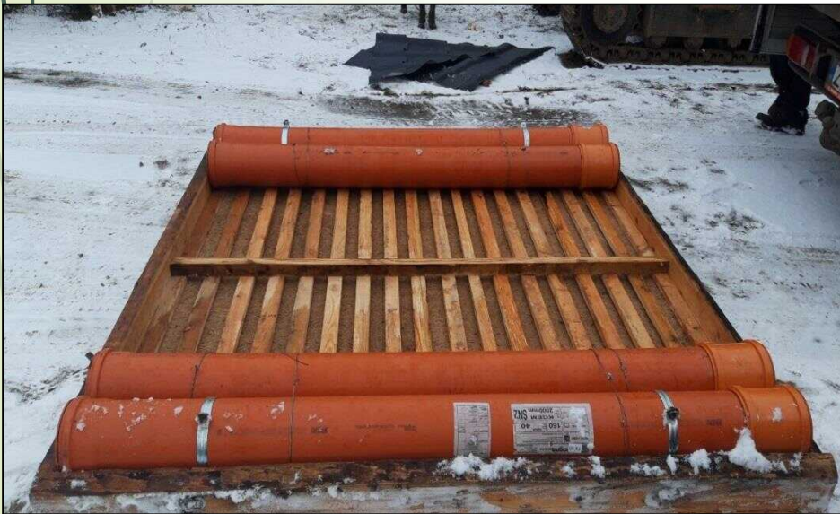
Floats made of plastic pipes (W. Spychała)
